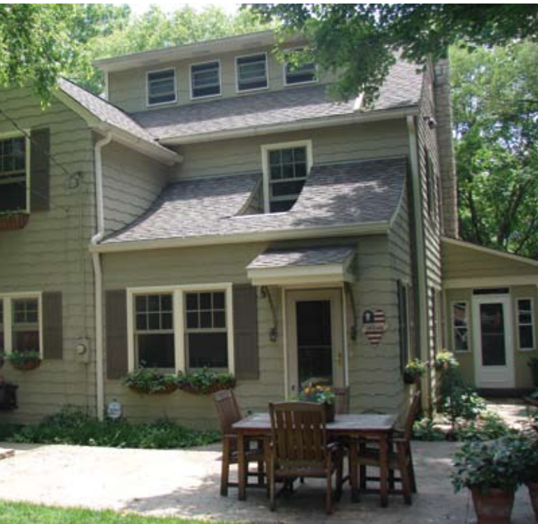
The addition's shed roof has a reverse dormer so that a second-floor window isn't obstructed.
